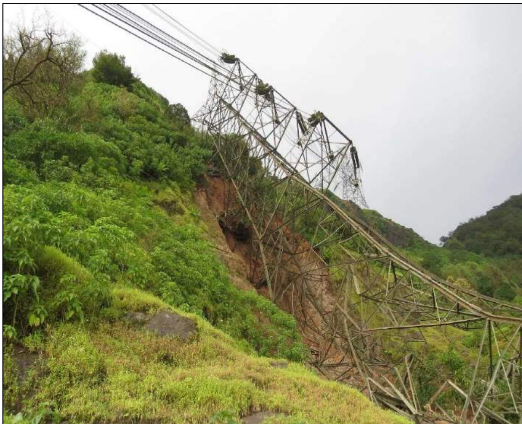
Collapsed tower no 150 (Jaigad-Karad line)
