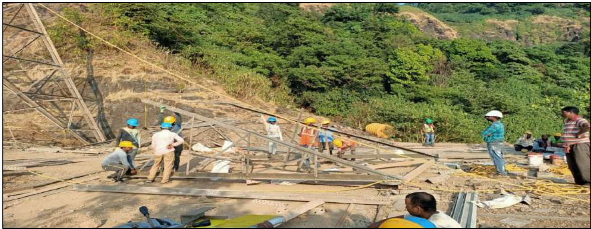
(Images: Cross arm assembly at Ground)
