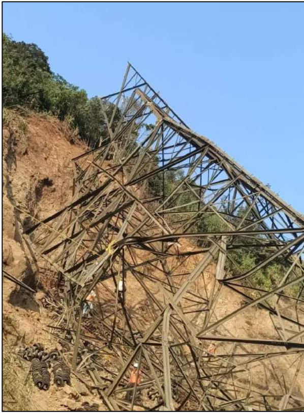
(Images: Tower dismantling by gas cutting)
