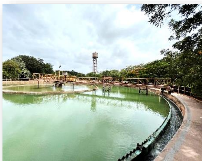
Raw water Treatment Plant-1
