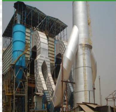
Ground De-dusting of CO - 3 2.3 lakhs m3/hr (2)
