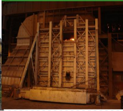
Cast House Fume Extraction at BF3 – 9 lakhs m3/hr (2)
