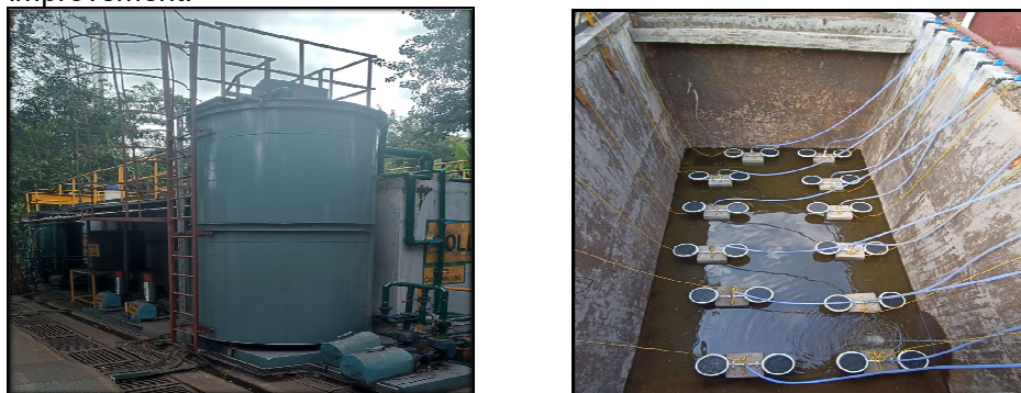
Plant STP Revamping
