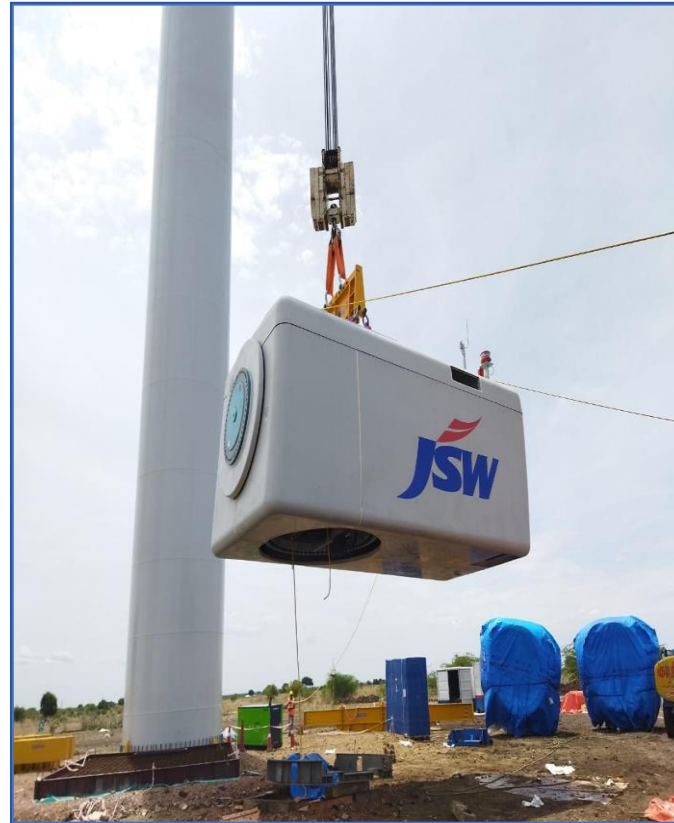
Nacelle Erection work in progress
