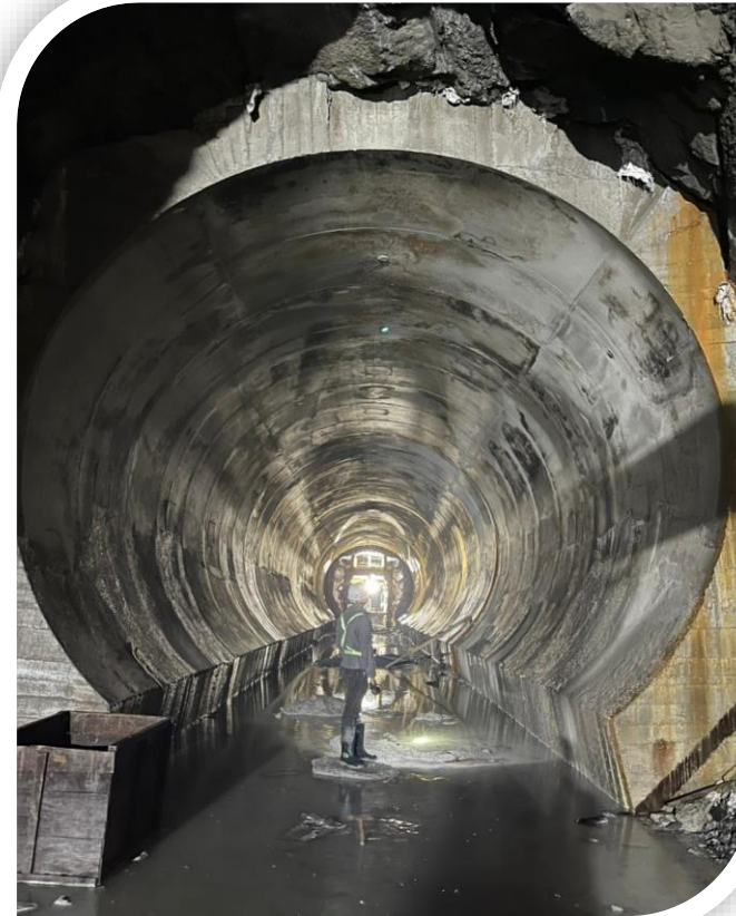
HRT Gantry Concrete Lining
