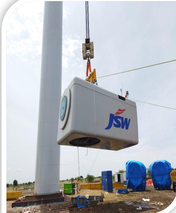
Nacelle and WTG erection
