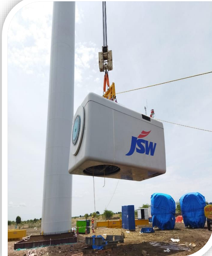
Nacelle and WTG erection
