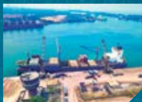
Mangalore Coal & Container Terminal, Mangalore, Karnataka
