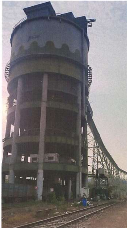
Silo loading attached with pipe conveyor
