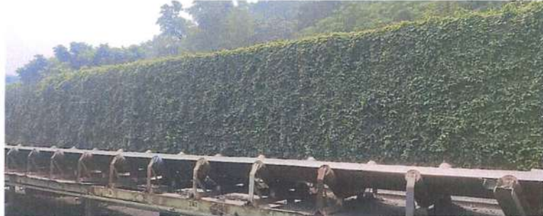
vertical garden across periphery
