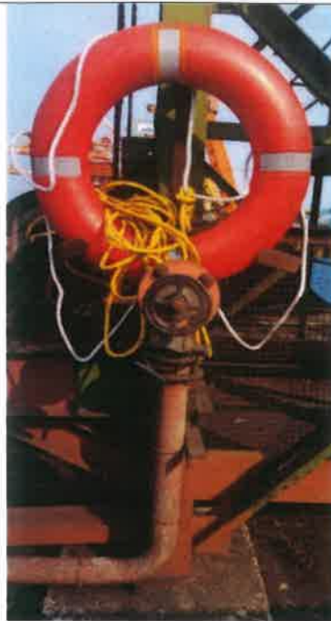
Fire hydrant post
