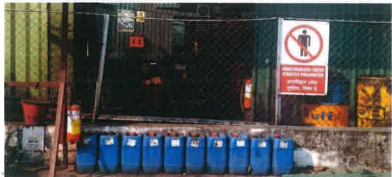
200 liters of Foam making compound, sand buckets & extinguishers
