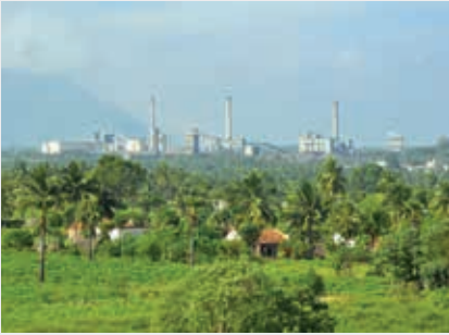
View of the Salem plant
