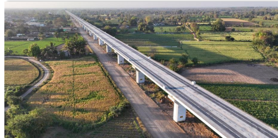
MAHSR Viaduct at Anand District, Gujarat
